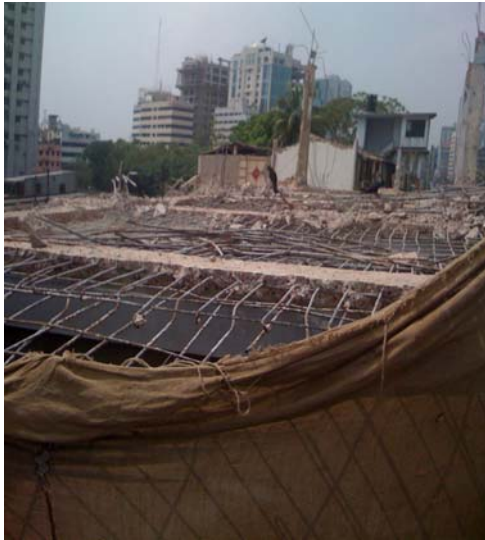
Figure 1 Demolition of Slab in progress
