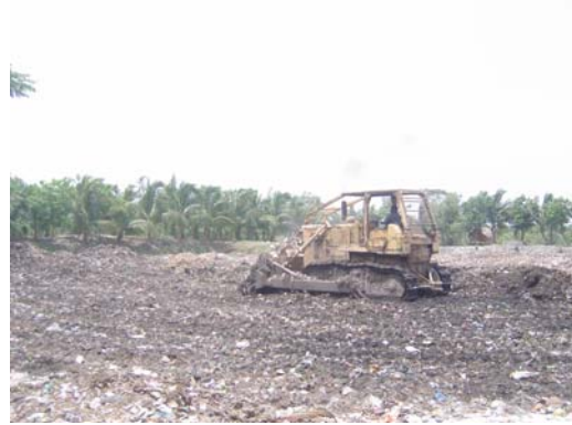
Figure 9 Waste spreading and compaction operation at the PSSL
