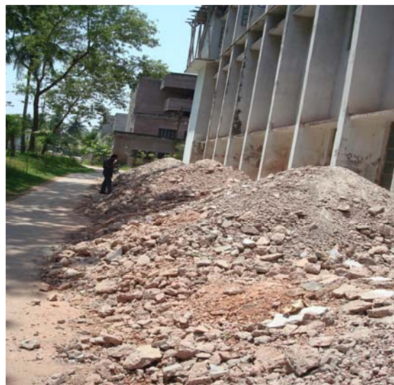
Figure 6 Storage of C&D wastes
