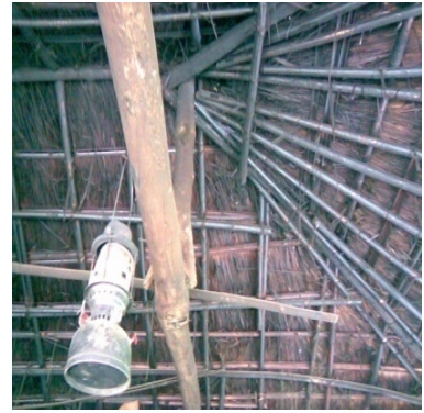
Figure 27 Bamboo beams & thatched roof
