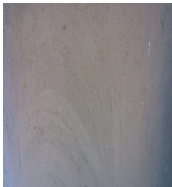
Fig. 20 Floor cladding with Dung & Husk
