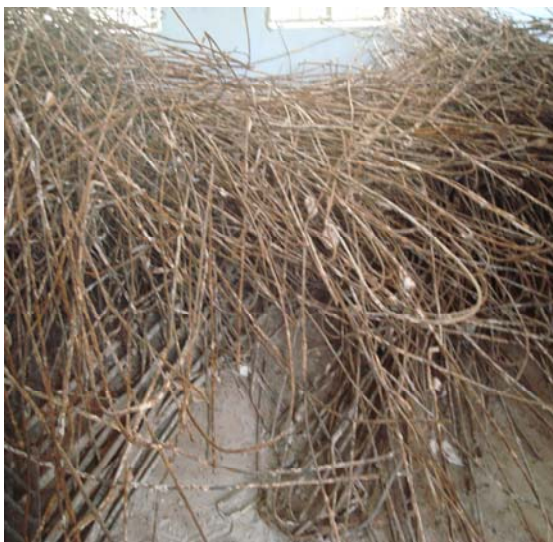
Figure 5 MS bars from demolished slab
