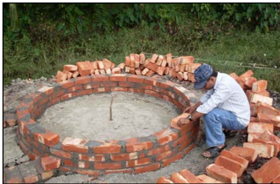
Figure 4 Construction of LFL treatment bio filter
