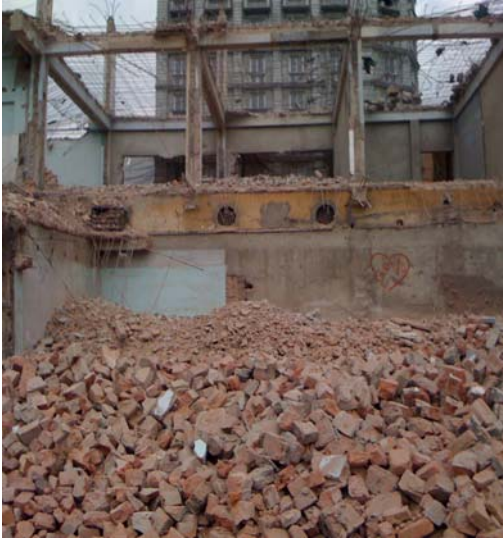
Figure 3 Demolition of brick works
