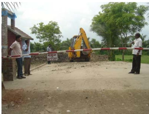
Figure 5 Control and inspection gate of incoming solid waste in the PSSL
