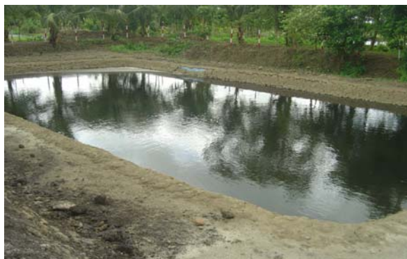
Figure 12 Leachate treatment pond in the PSSL Figure 13 Leachate reservoir pond in monsoon
