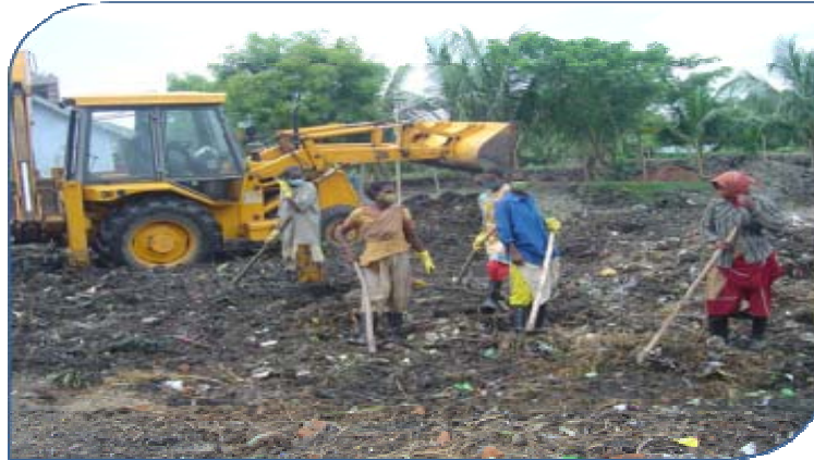
Figure 2 Landfill operations by the workers
