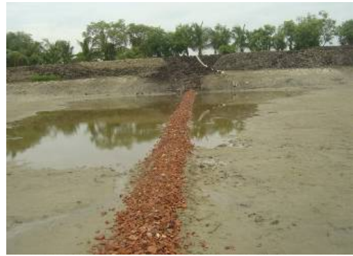
Figure 13 Leachate collection pipe with brick aggregates as filter media
