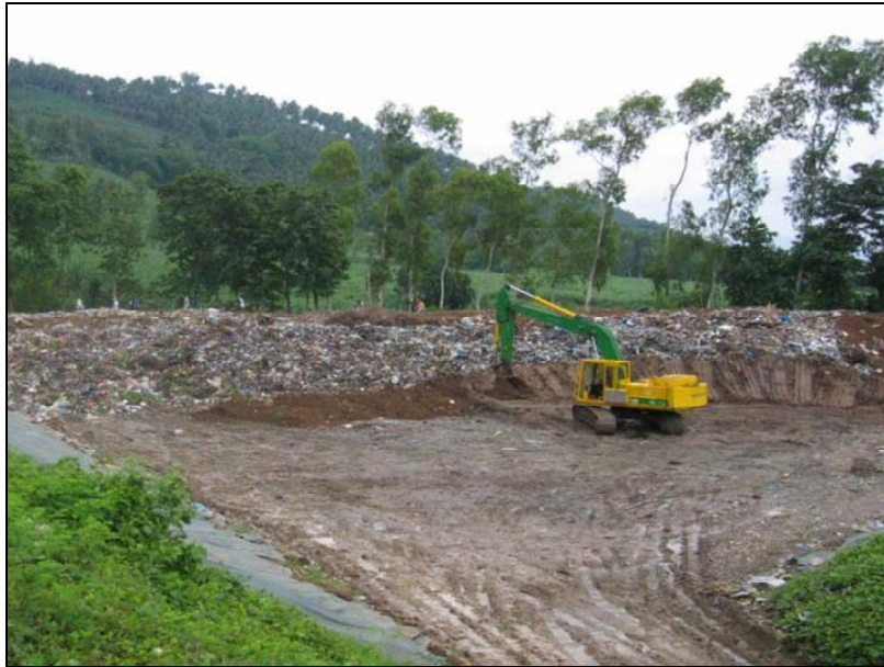
Figure 4 Waste compaction and soil coverage at the landfill Bais City in 2004
