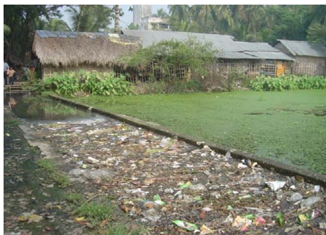
Figure 1 Situation of a drain due to throw out of waste
