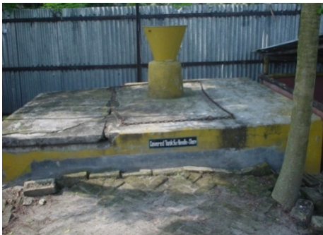
Figure 10 Concrete Chamber to store Sharp
