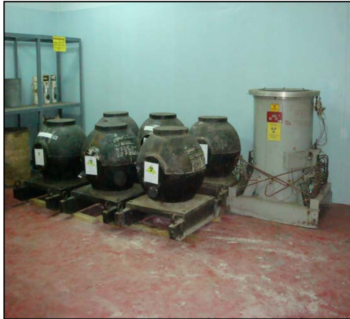
Figure 1 Spent sealed source room
